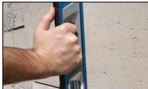
Use a large level to check and maintain an even-face plane over multiple tiles.
